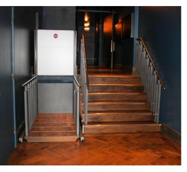
The FlexStep stairlift is designed to function both as an ordinary staircase and as a wheelchair lift. Developed and manufactured by Liftup, the FlexStep is flexible and equally useful for pedestrians and wheelchair users alike.
